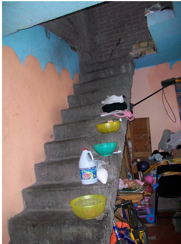
Figure 5. Interior staircase to third floor which required forcing a new opening in the concrete ceiling of the second floor. Isidro Fabela colonia, Mexico City.
