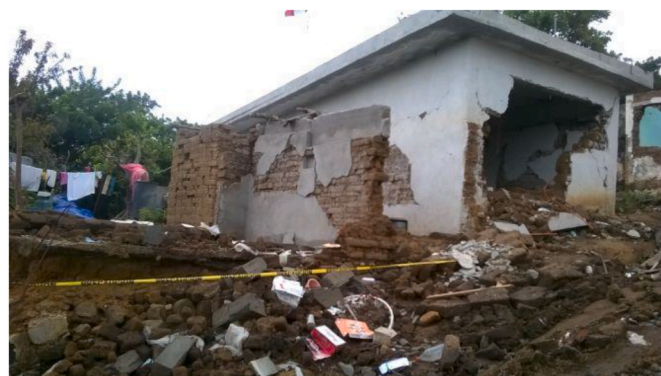
Fig. 4. Earthquake damage to consolidated adobe walled house (Image taken by Alejandro Luna López).
