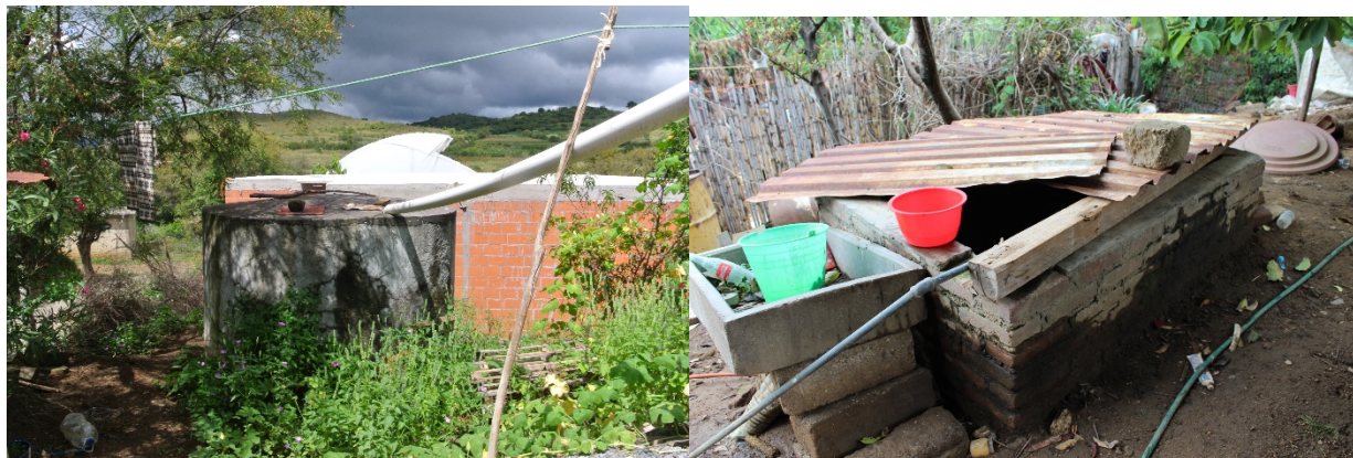
Photograph 4.2 (left): Roof-fed Rainwater to Storage Tank SFX. Photograph 4.3 (right): Water storage tank in San Fco. Xochiteopan. Note the feeder in-pipe, as well as buckets to scoop water for washing etc. (Images taken by Dr. Peter Ward).
