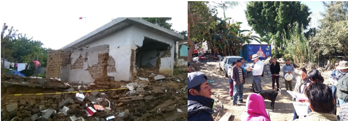
Photograph 4.4 (left): Earthquake damage to consolidated adobe walled house (Image taken by Alejandro Luna López). Photograph 4.5 (right), Members of the FCP on site to discuss plans for new homes with Doña Francisca's family (see also Appendix. 4 Case 2a https://lahn.utexas.org/Puebla/App4.html ) (Image taken by Alejandro Luna López)
