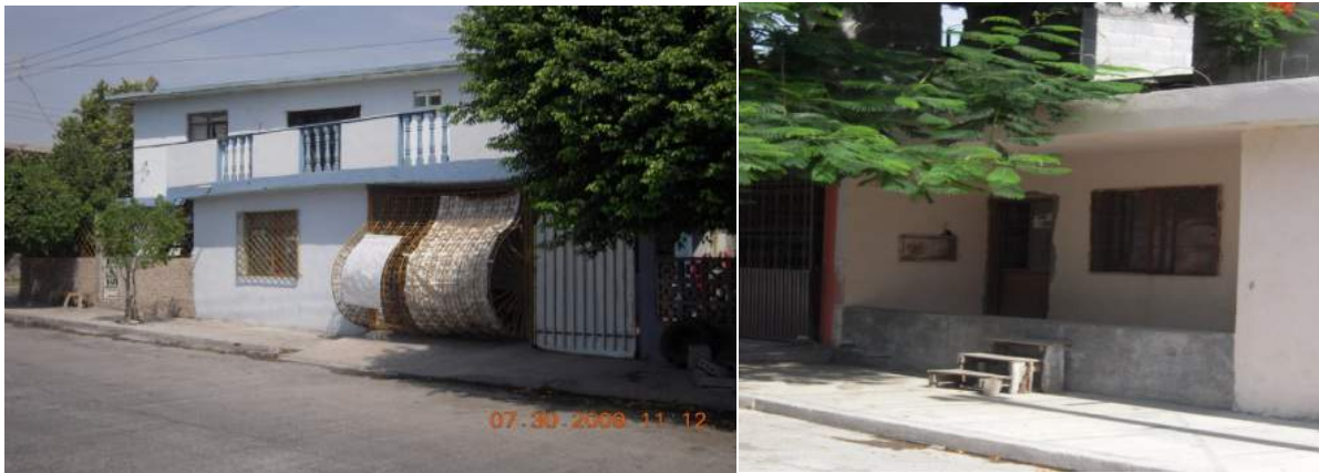
Photo 4.3 (left) “Pregnant” garage doors provide room for vehicles; Photo 4.4. (right) Front of house barrier to reduce inundation after flooding
