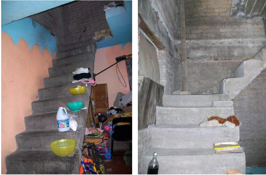
Photos 4.9 and 4.10. New staircase in the Toribio Home
