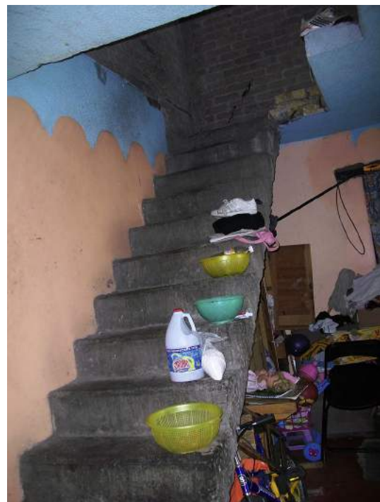
Fig. 5. Interior staircase to third floor which required forcing a new opening in the concrete ceiling of the second floor. Isidro Fabela colonia, Mexico City.
