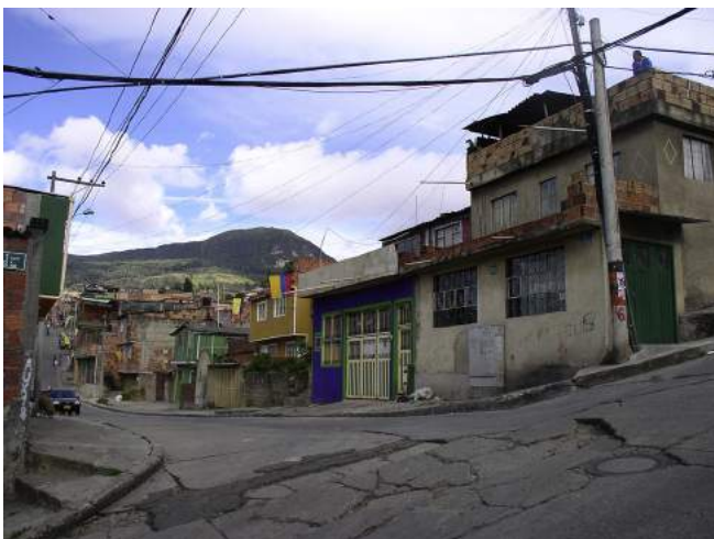
Fig. 7. Street view of barrio Atenas in Bogotá showing different levels of deterioration and distress of the street and infrastructure.
