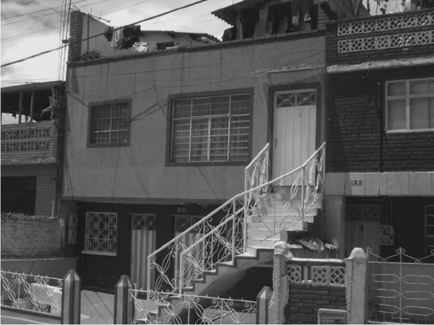
Figure 2B 2008. Staircase access to second story dwelling. Note two dwellings on ground level. Shared space is the front patio. Guadalajara.
