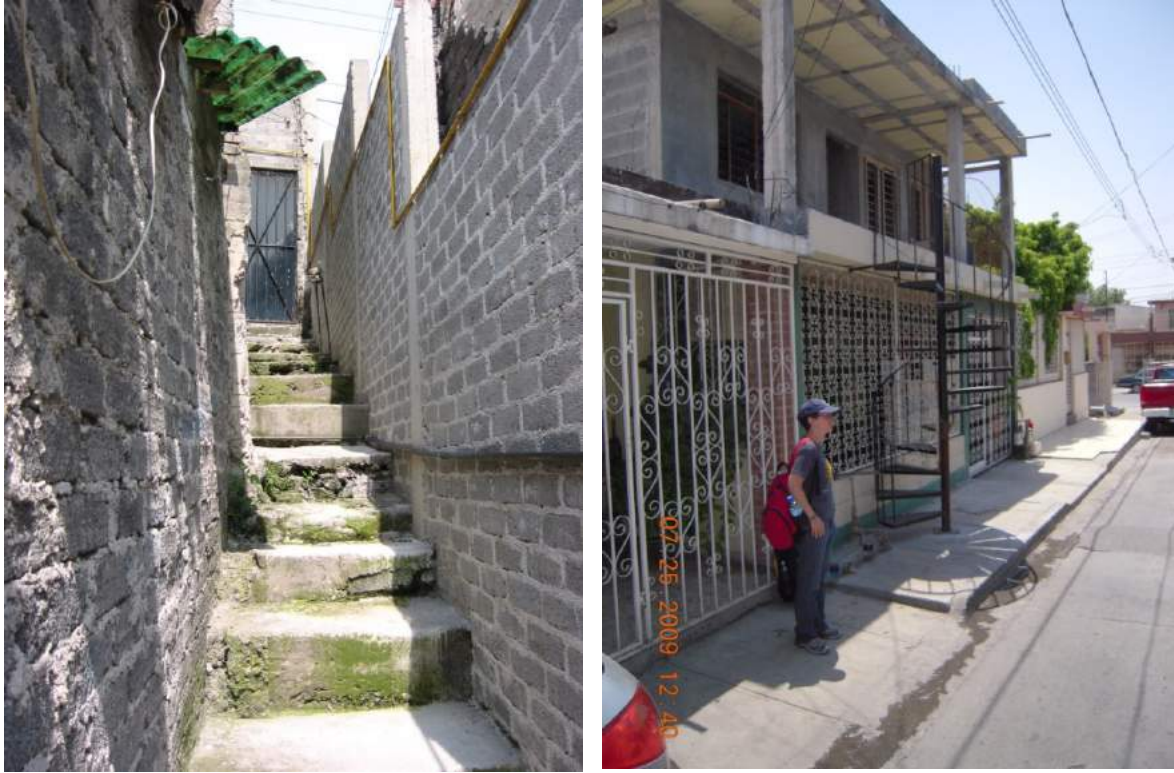
Photo 2.3. (left) Side access to rear dwellings in Isidro Fabela, Mexico City. Photo 2.4. (right) Stairs from sidewalk to room rental above Valle Santa Lucia, Monterrey. Note the conversion of room to a garage with sliding door and how stairs and door impede the window.
