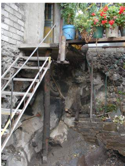
Photos 12.13 and 12.14. Problems with structural conditions. Photo 12.13 (left) shows a foundation and stone support for the metal stairs that is provisional and insecure. Photo 12.14 (right) shows a roof without adequate waterproofing that has allowed damp to break through the ceiling in most of the rooms so that the roof is in danger of collapse.
