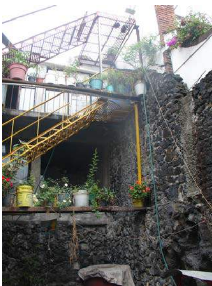
Photos 12.15 and 12.16. Problems with structural conditions. Photo 12.15 (left) shows a stairway that is unsafe and lacks adequate support. Photo 12.16 (right) shows a railing that is unsoldered at various points with wide gaps between the bars. There are also gaps in the floor near the railing, making it especially dangerous for a three year old and her mother if they lean over the railing to hang out the washing.
