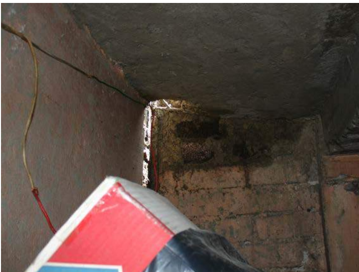
Photos 12.13 and 12.14. Problems with structural conditions. Photo 12.13 (left) shows a foundation and stone support for the metal stairs that is provisional and insecure. Photo 12.14 (right) shows a roof without adequate waterproofing that has allowed damp to break through the ceiling in most of the rooms so that the roof is in danger of collapse.
