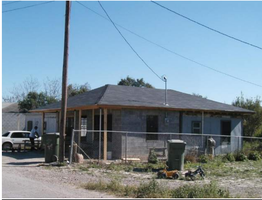
Figure 1.2. Typical self-help building in Starr County. (Note original house at rear serving as a temporary dwelling.)
