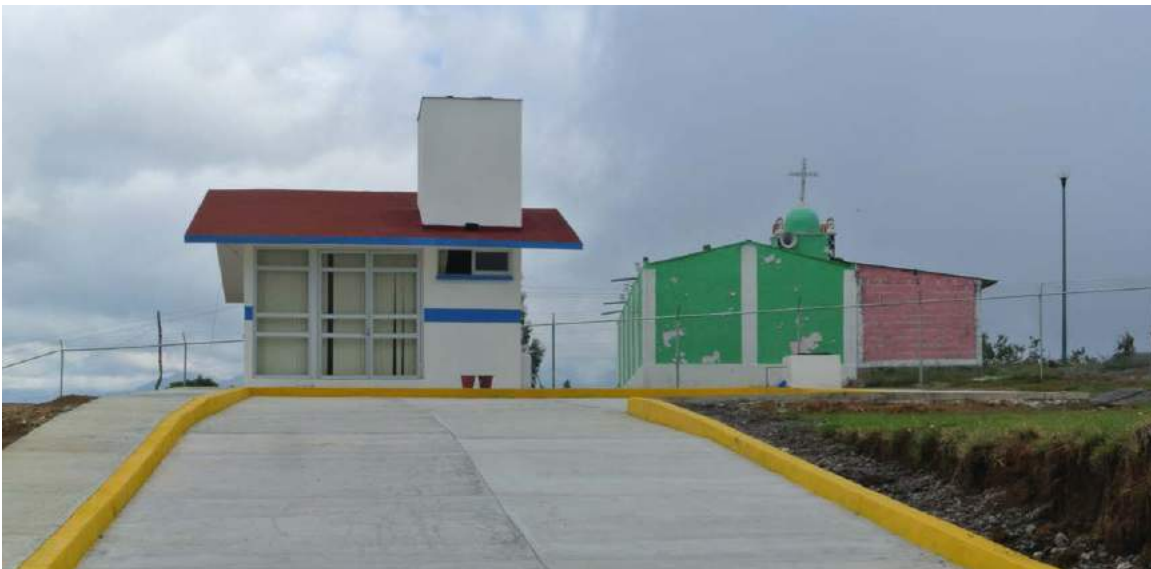
Photograph 2.4: The picture above is the new Casa de Salud constructed during August 2019 and finished in early October of 2019. The structure was built by government contractors and replaced a cinderblock room that was created after the Earthquake in 2017 (Image taken by Dr. Peter Ward, October 2019).
