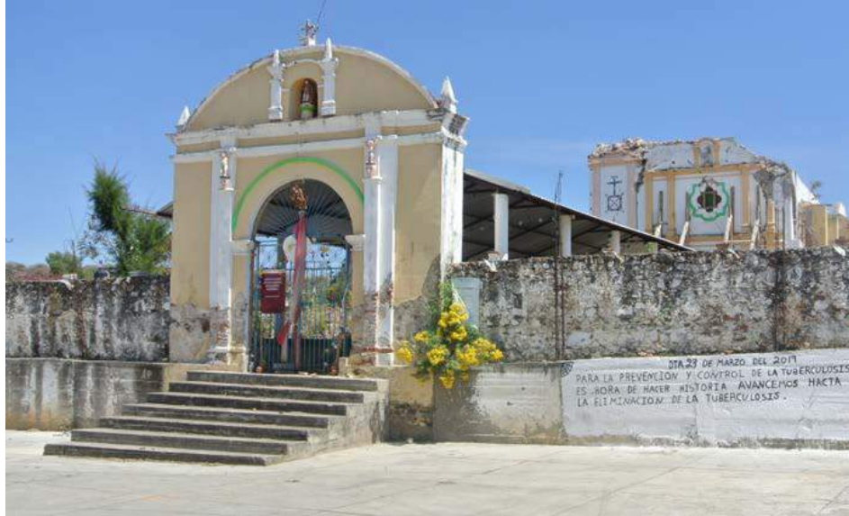
Photograph 1.5: Town church deeply affected by the 2017 earthquake (Image taken by Dr. Peter Ward).
