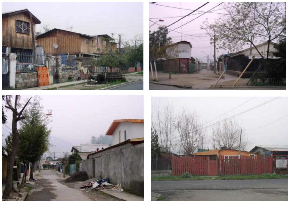
Photos 9.1 – 9.4. Photos of El Bosque, showing narrow side streets and wooden one- and two-story self-help dwellings.
