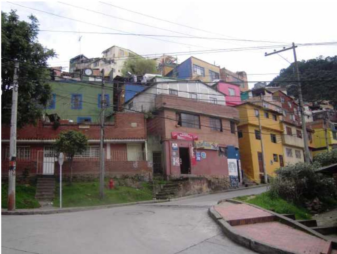
Photo 7.3 Damage and discontinuity of sidewalks in Barrio Casa Blanca (Photo by Peter Ward)
