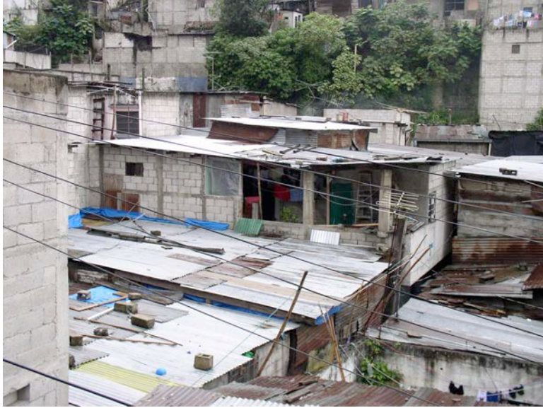
Photo 1.2. Dilapidation and intensive use, El Esfuerzo, Guatemala City.
