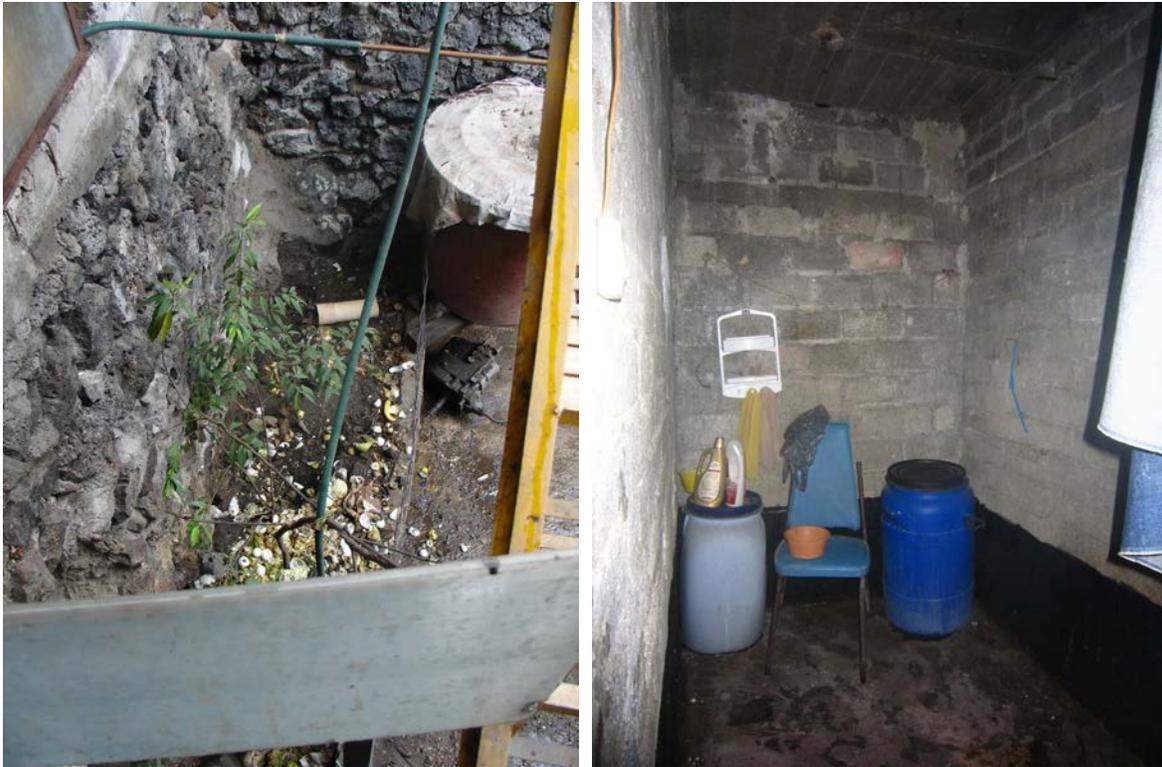
*Photos 12.17 and 12.18. In Photo 12.17 (left) gas pipes (covered in green) cross over each other with a water tank below. The gas pipes are not attached to the wall. Each tenant makes his or her own installation and connection. Photo 12.18 (right) shows a common shower space. There is no actual shower; residents wash from buckets.*
