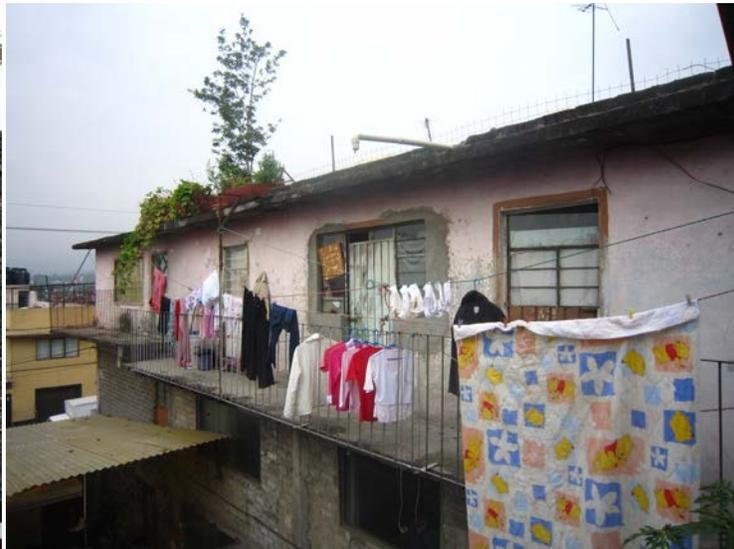
*Photos 12.15 and 12.16. Problems with structural conditions. Photo 12.15 (left) shows a stairway that is unsafe and lacks adequate support. Photo 12.16 (right) shows a railing that is unsoldered at various points with wide gaps between the bars. There are also gaps in the floor near the railing, making it especially dangerous for a three year old and her mother if they lean over the railing to hang out the washing.*
